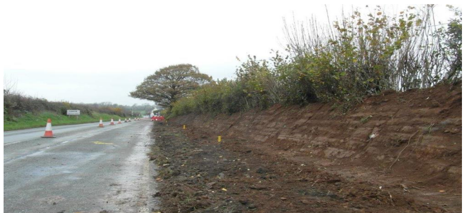
Figure 7. Hedgebank following incremental dragging to widen a section of road for health and safety to implement a new footpath. Road widened to the retained tree in the distance and then the development continued on the opposite side of road.
